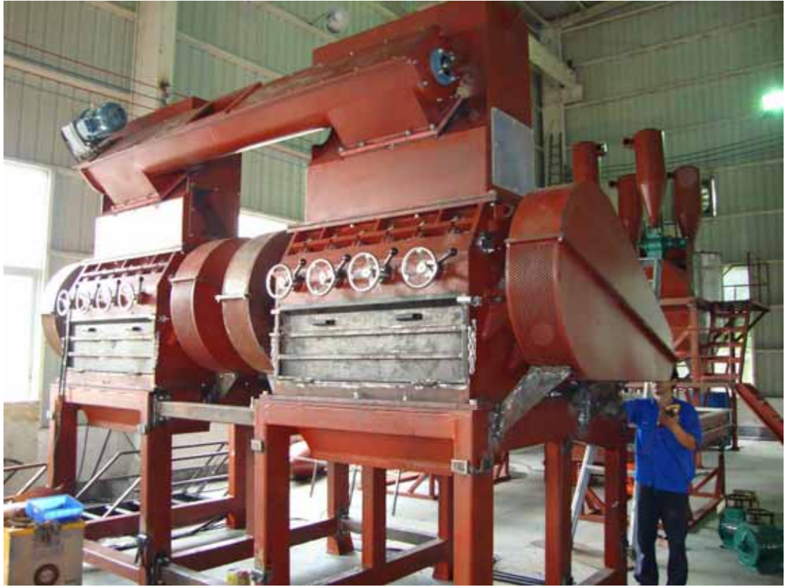
SETUP VIEW OF SECONDARY RASPER GRINDERS IN SYSTEM
